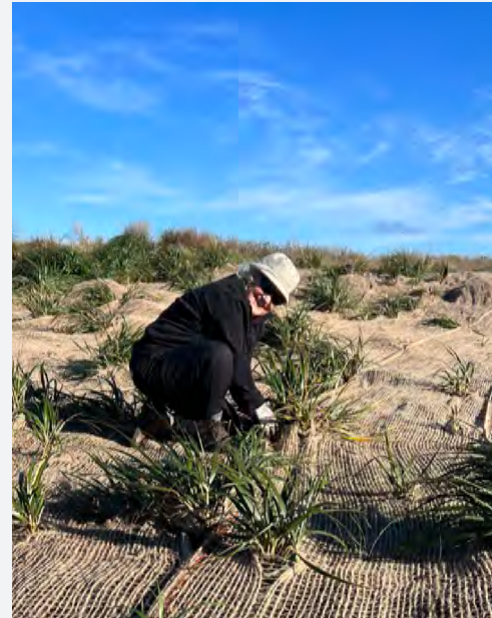
Following seeding, laying and pinning of jute, Kathy pulls the existing dune grass through the open and flexible weave. Seedlings and new plants will grow up through the jute fabric, which will decay within a few years' time.
